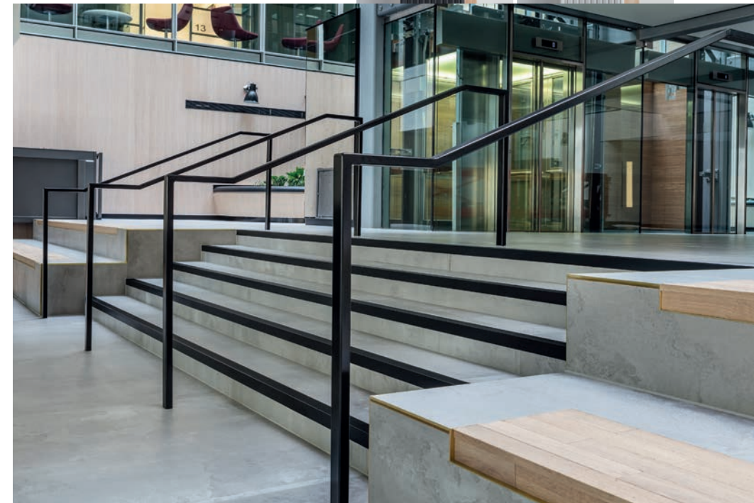
Below: Premium CMS black anodised nosings with stone flooring, London, EC4
