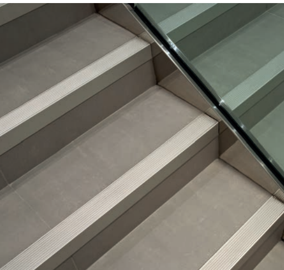
Right and bottom right: Premium CMS black anodised nosings with stone flooring, London, EC4
